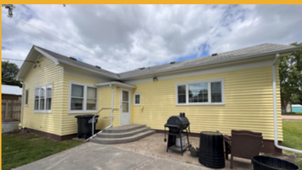
Home Rehab Project
